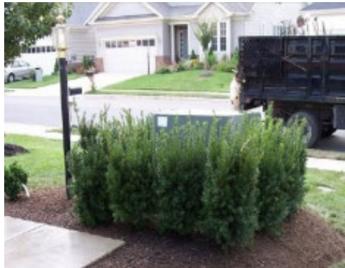
Utility boxes should be screened by taller growing plants.
