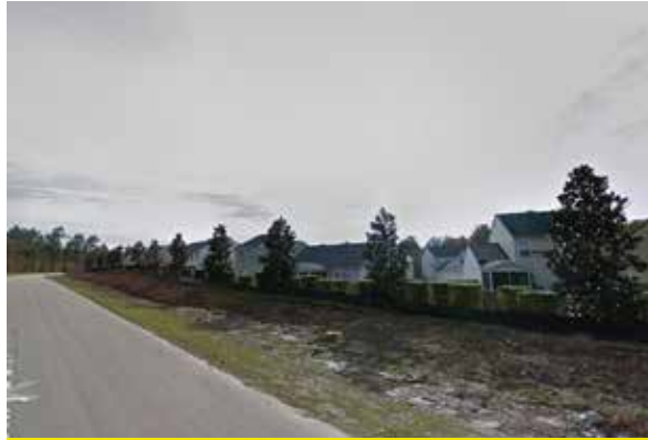
Location of planned shared-use path on Henry E. Brown, Jr. Boulevard as part of roadway widening project.
